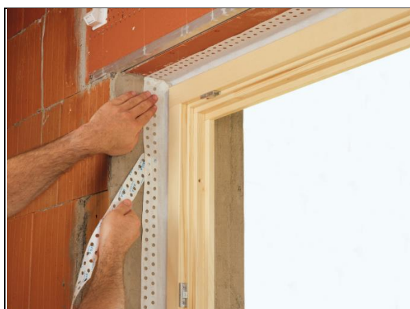
Figure 1 Internal window — corner detail
