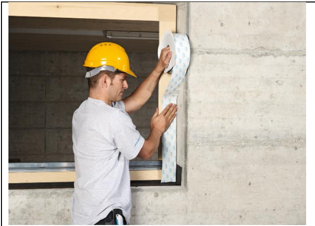
Figure 4 Installing tape vertically
