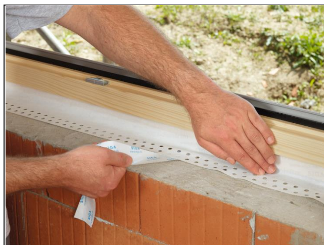
Figure 2 Removal of release film
