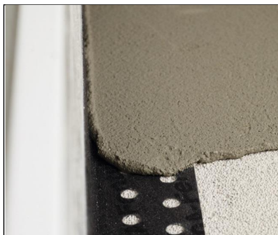
Figure 6 Application of plaster
