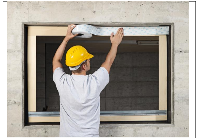
Figure 5 Installing tape at top of frame
