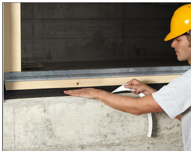
Figure 3 Installing tape at bottom of frame
